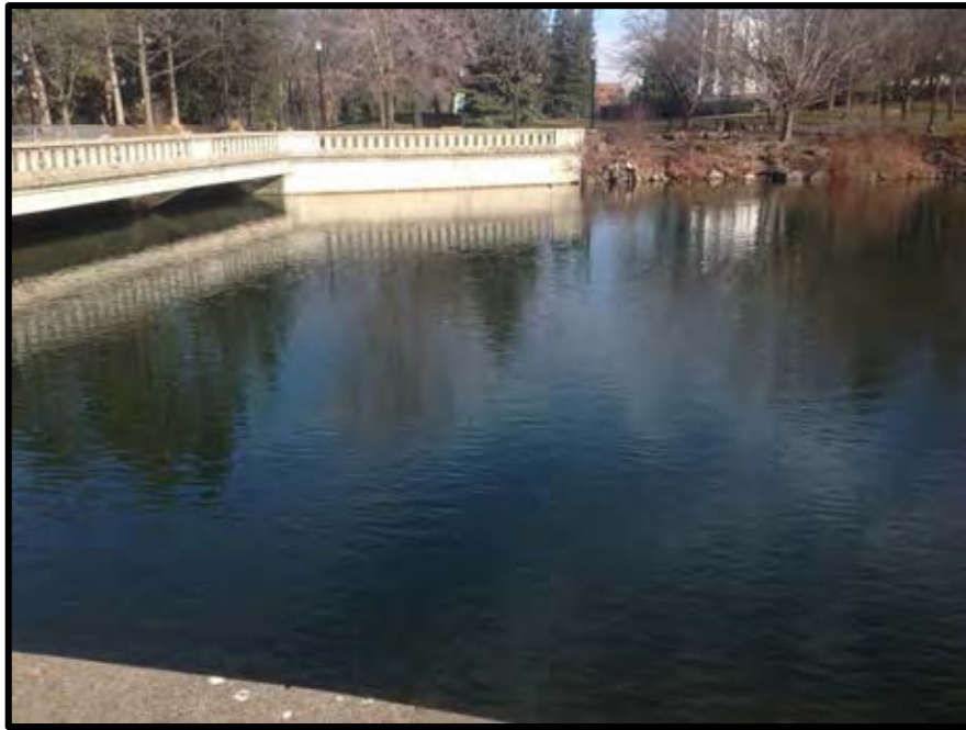
Photograph 2. General view of the South Howard Street Bridge (facing northwest).
