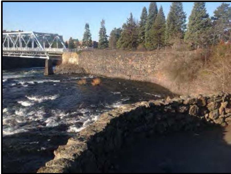
Photograph 7. General view of the North Howard Street middle bridge (facing south).
