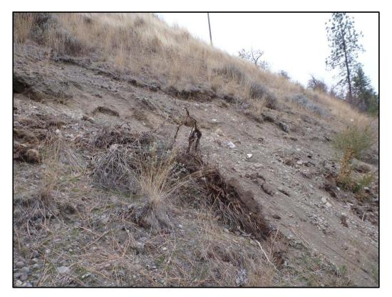
Photo 4: Eroding slope at west end of project area where proposed slope break planting structures are proposed.
